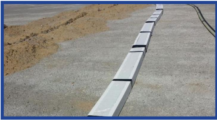
Insulating supply lines using EPS
